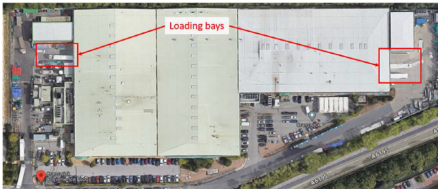
Fig. 4. Satellite photo of Cranswick Convenience Foods, South Yorkshire, S73 0UN (factory site) with loading bays indicated.
